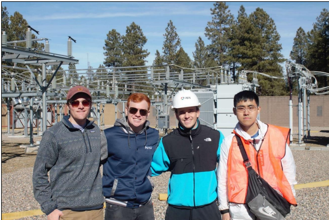
Figure 1: APS Soldier Pass substation tour team photo. Pictured (left to right): Trevor Senior, Evan Higgins, Winston Steele, and Zonghua Ouyang.
